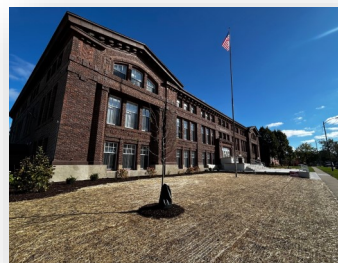
The restored façade and landscaping of the original Belvidere High School
