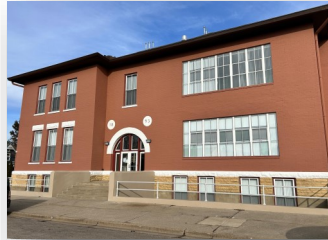
Exterior photo of the Annex Building at Pearl Place Apartments
